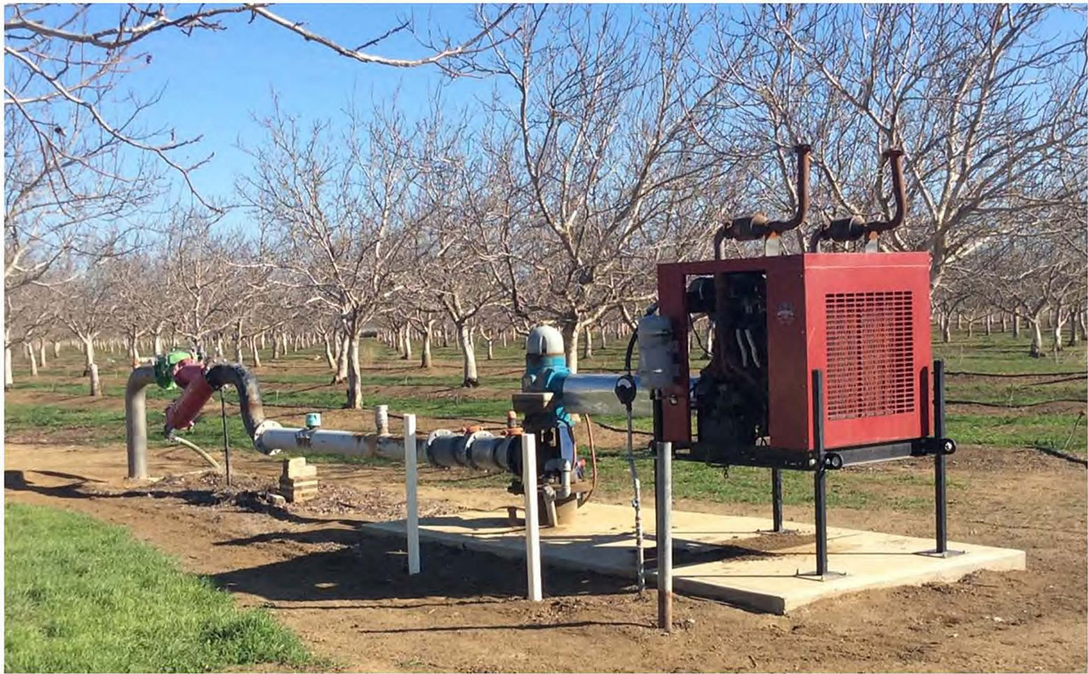
SINGLETON ORCHARD PROPANE POWERED WELL
